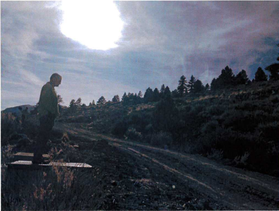
Power and Telco
